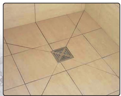
Varme Offset Shower Tray (pre-grout). Tiles cut to follow pre-made fall.
